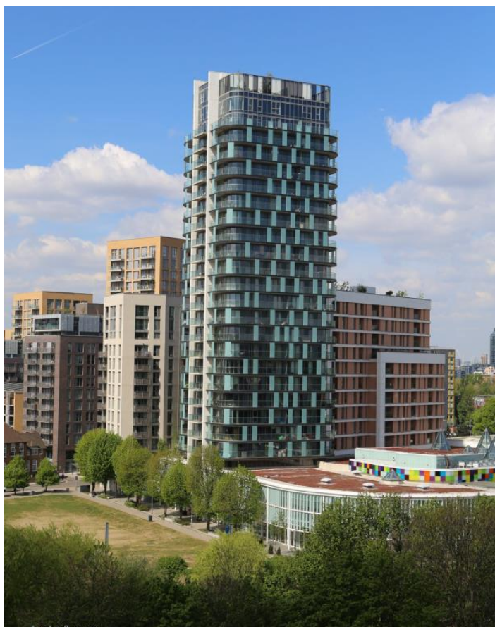
Figure 9.9: A recent mixed use development in Lewisham
