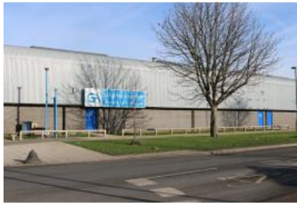
1 - Blank frontages on Surrey Canal Road
